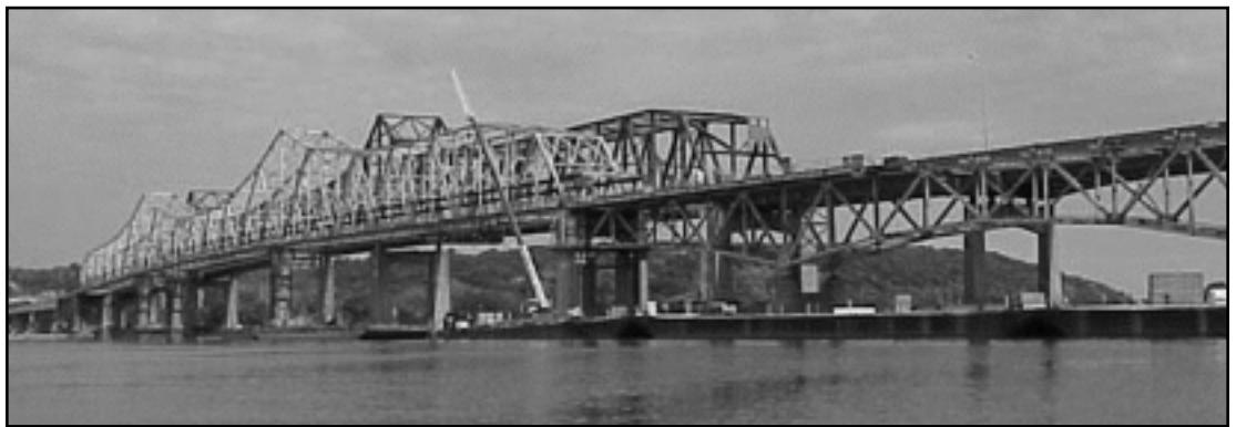
The McClugage Bridge—carrying US 150 and US 24 over the Illinois River, Peoria, Illinois
