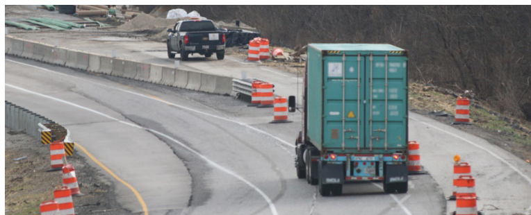
Figure 3. Photo. Lane shifts within horizontal curves can be difficult for commercial motor vehicle drivers to navigate.
