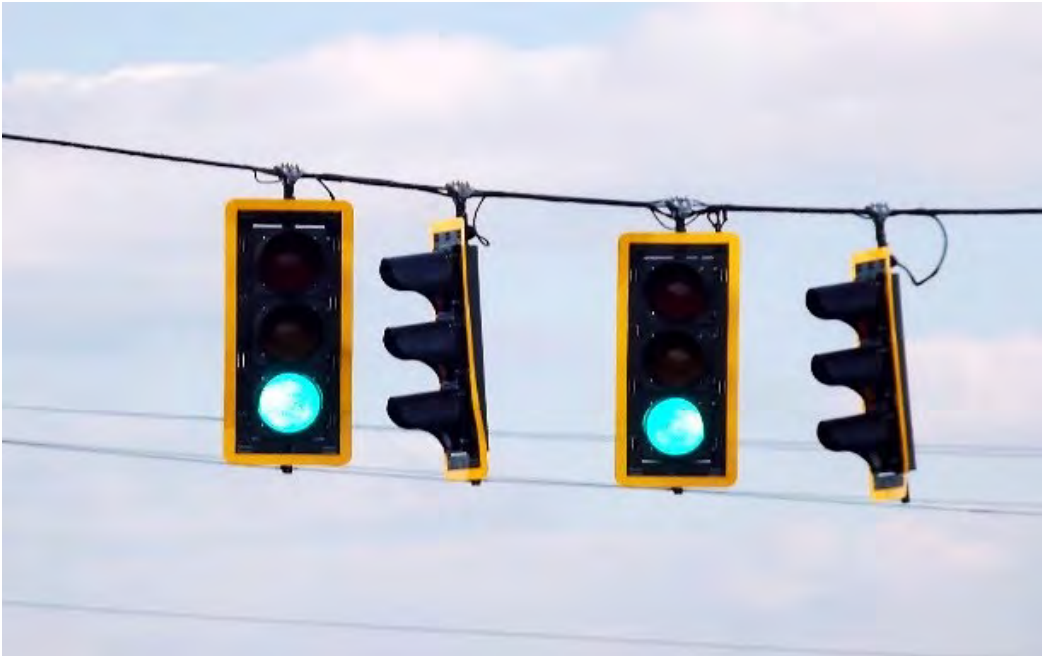
Figure 11. Photograph. Traffic signal indication with a solid backplate.
