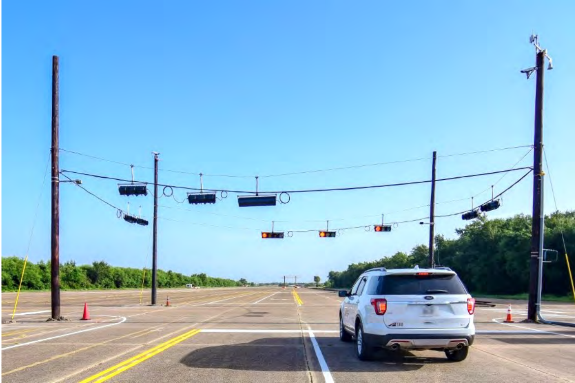
Figure 16. Photograph. Example of a span wire installation.
