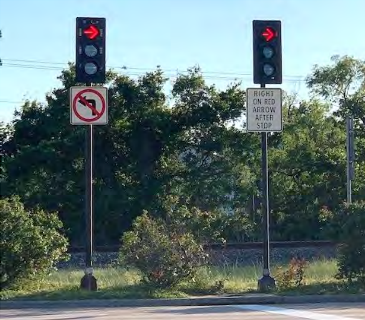
Figure 17 Photograph. Example of pedestal-mounted traffic signal.
