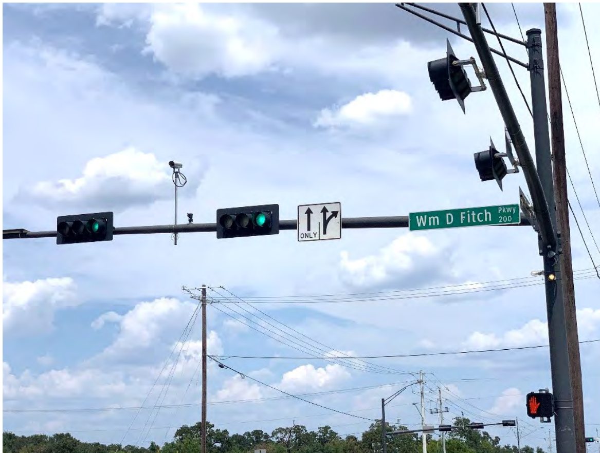
Figure 15. Photograph. Typical mast arm traffic signal installation.
