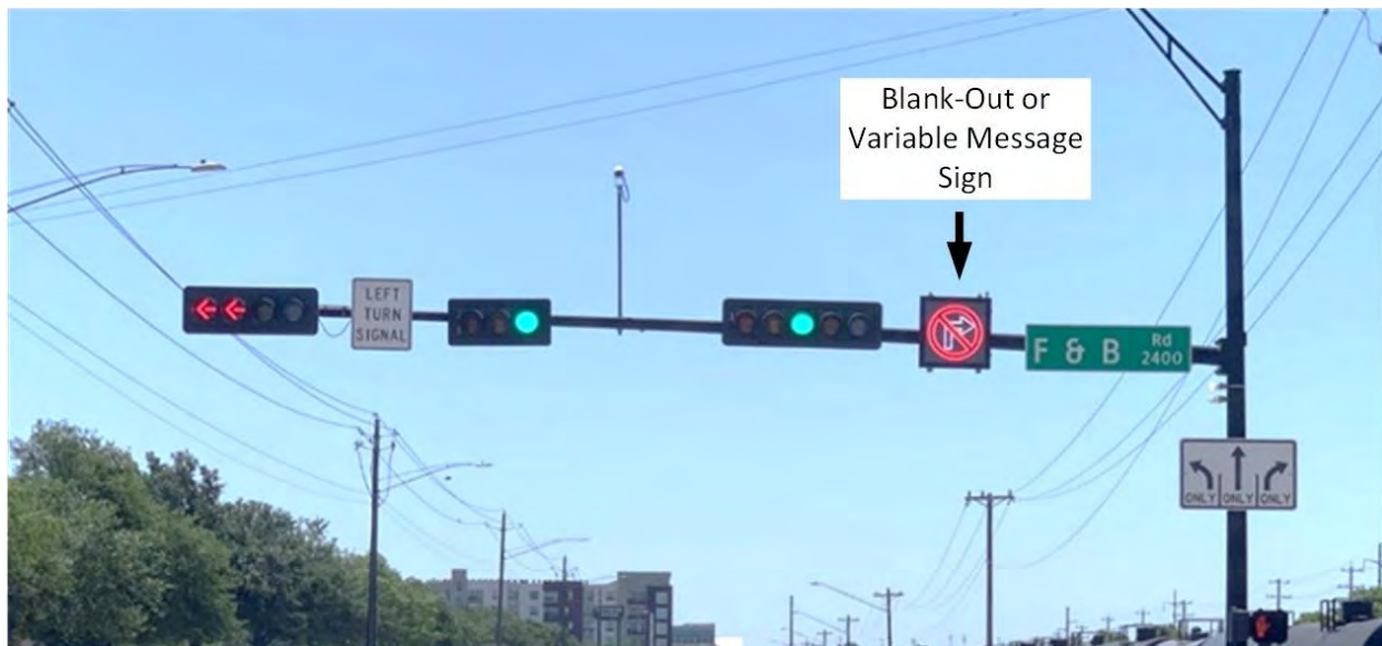
Figure 35. Photograph. Example of blank-out sign operated by a traffic signal.
