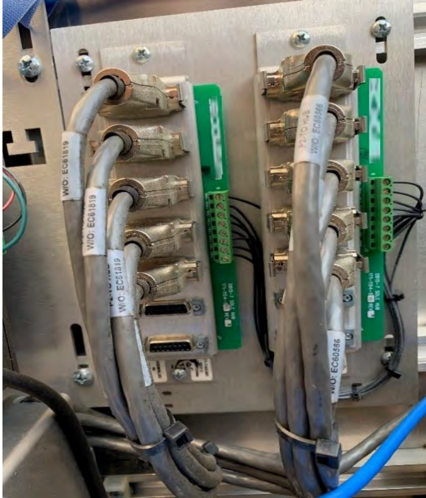
Figure 32. Photograph. Example of a BIU hub in a TS2 traffic signal cabinet.
