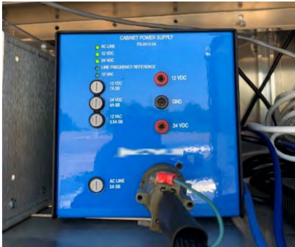
Figure 27. Photograph. Example of a power supply unit in a NEMA TS2 cabinet.
