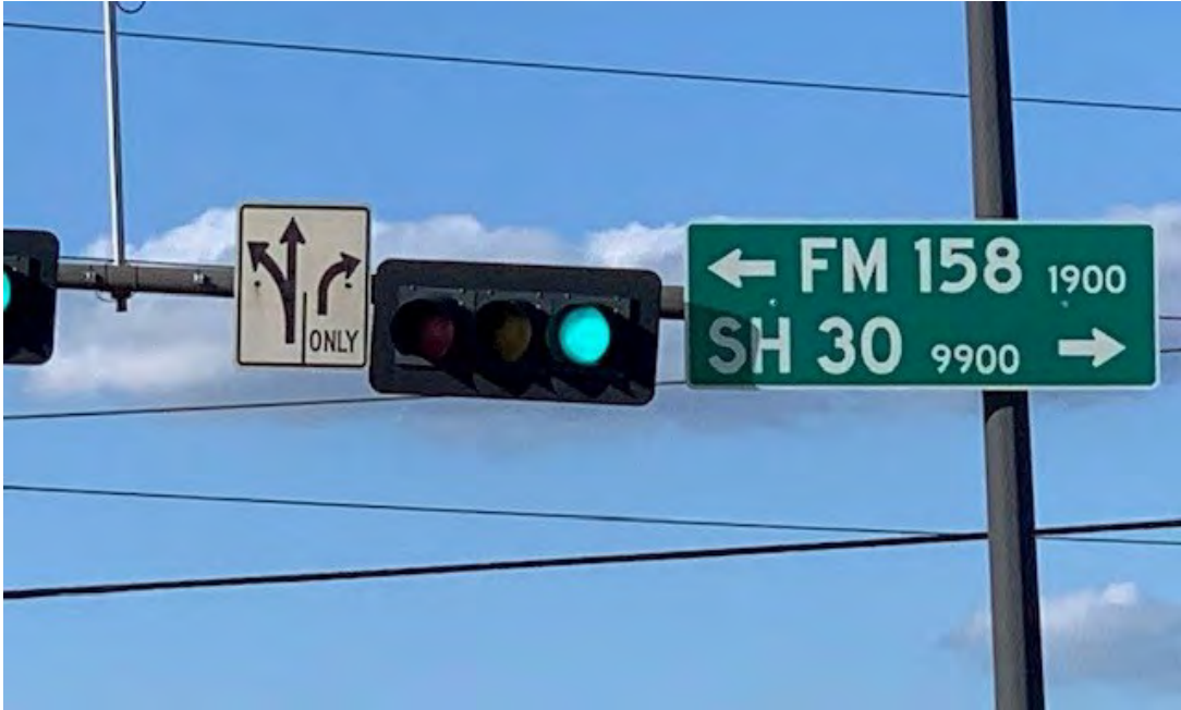
Figure 11. Photograph. Traffic signal indication with a solid backplate.
