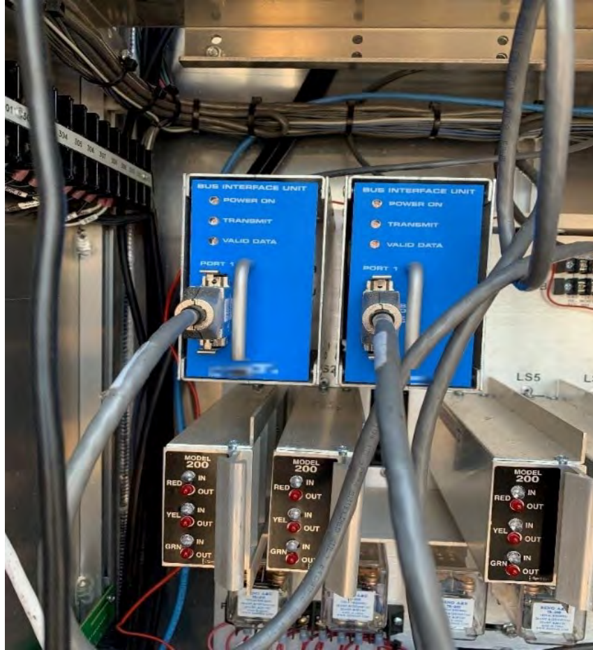
Figure 31. Photograph. Example of BIUs in NEMA TS2 traffic signal cabinet.
