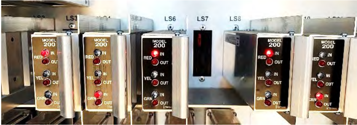
Figure 30. Photograph. Example of load switches in a NEMA TS2 cabinet.
