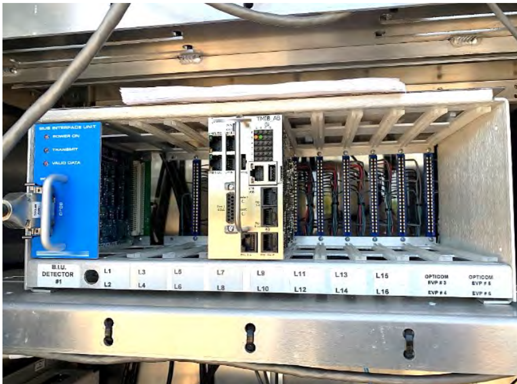
Figure 26. Photograph. Example of a rack-mounted detector input in a NEMA TS2 cabinet.
