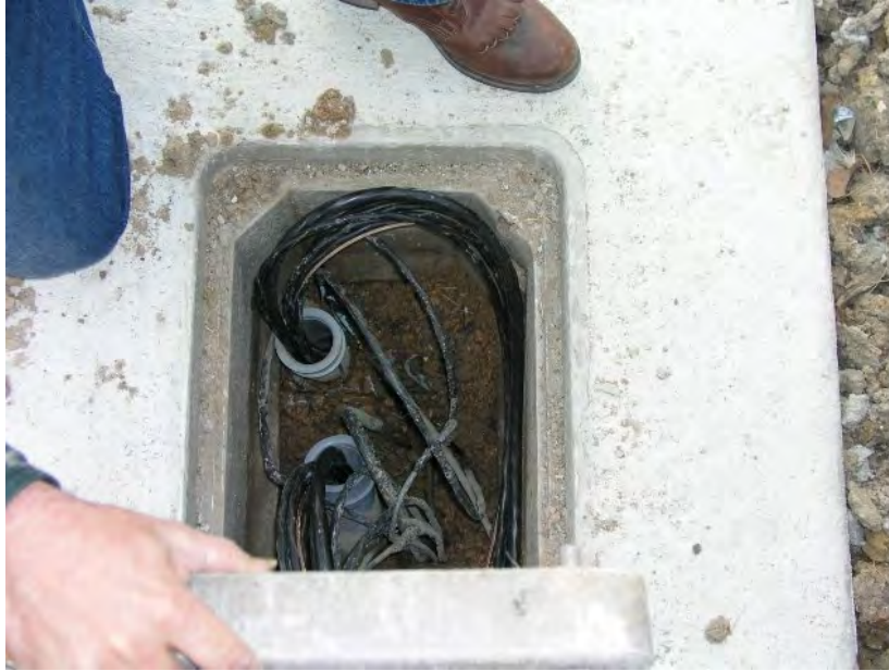
Figure 18. Photograph. Example of a ground box at a signalized intersection.
