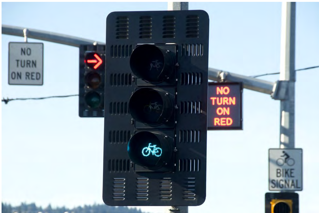
Figure 13. Graphic. Example of bicycle traffic signals at urban intersection.
