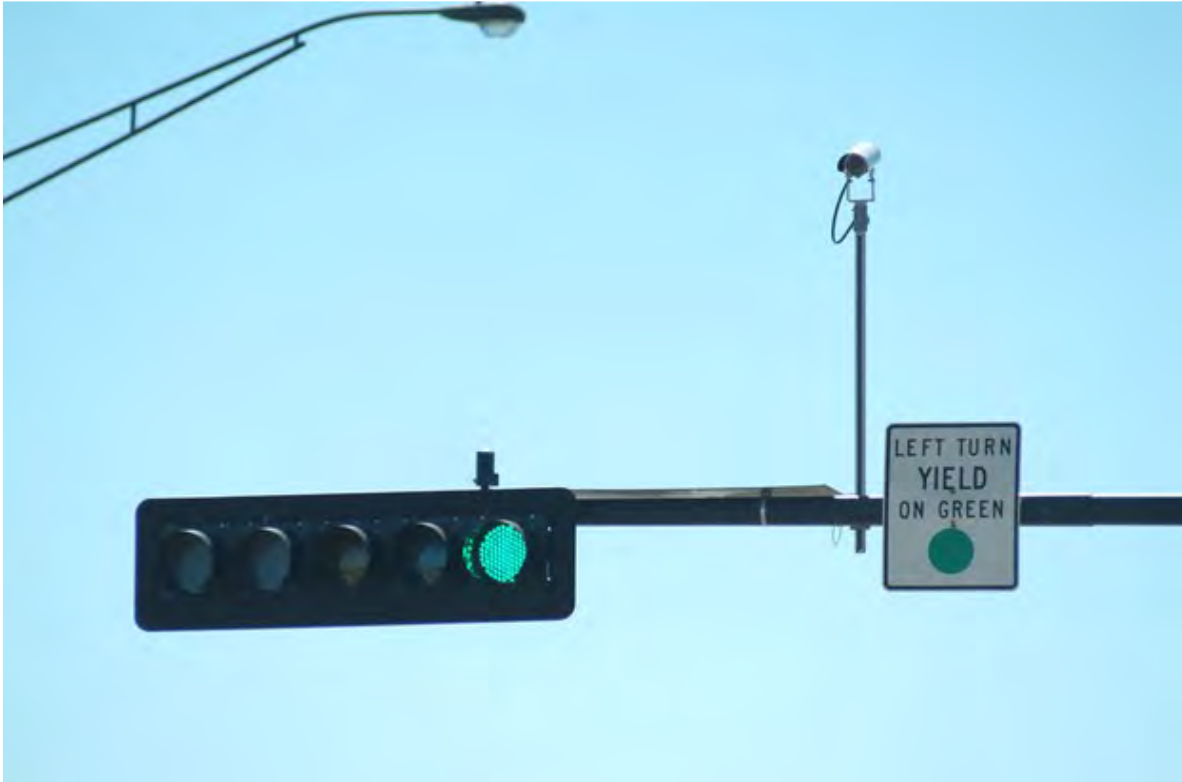
Figure 49. Photograph. Example of video detection cameras installed on traffic signal mast arm.
