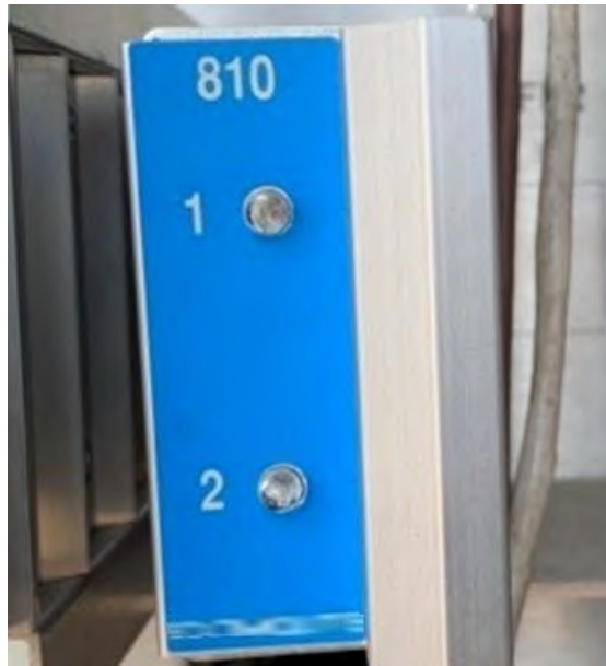
Figure 33. Photograph. Example of a solid-state flasher unit in a NEMA TS2 cabinet.
