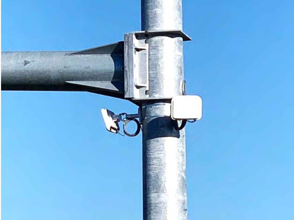
Figure 51. Photograph. Example of a microwave/radar sensor installed on a traffic signal mast arm.
