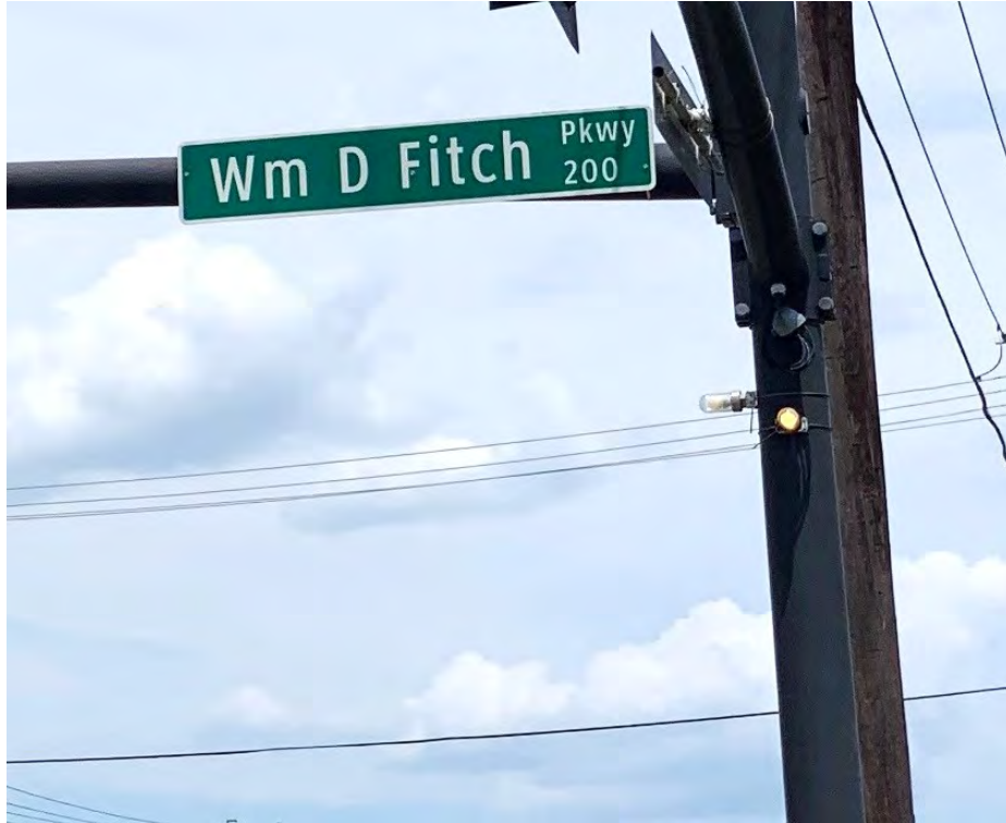
Figure 37. Photograph. Example of an enforcement light mounted to a pole at a mast arm installation.
