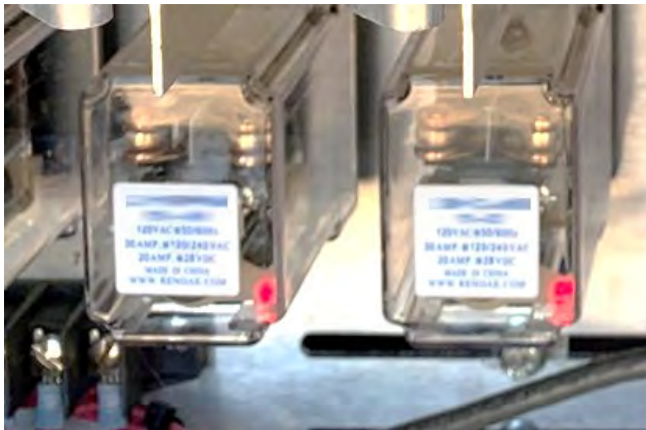
Figure 34. Photograph. Examples of flash transfer relays in a NEMA TS2 cabinet
