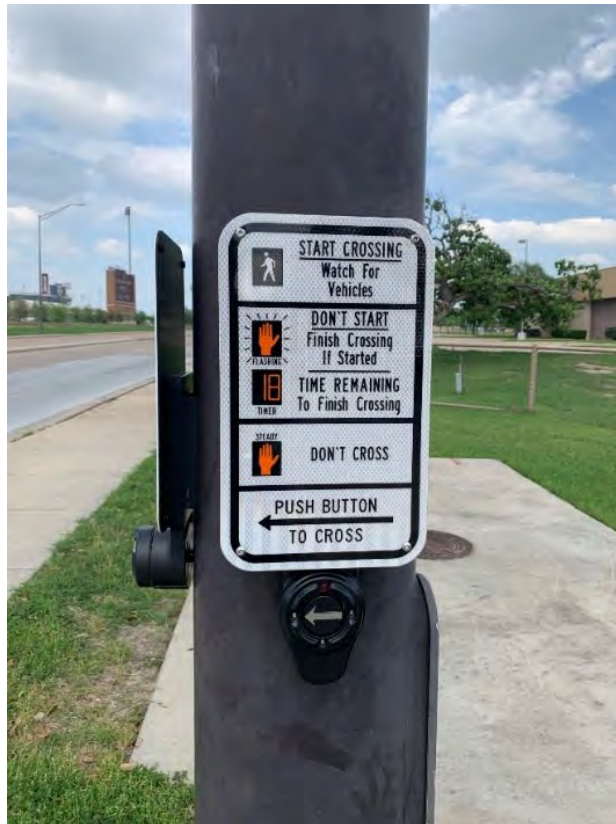
Figure 36. Photograph. Example of an accessible pedestrian signal installation.
