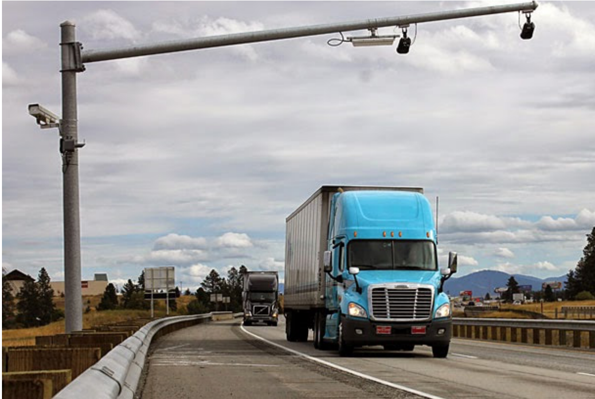
Figure 3.6. Example of a weigh-in-motion system.
