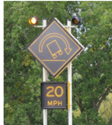
Figure 3.10. Minnesota Department of Transportation (MnDOT) Truck Rollover Warning System sign.
