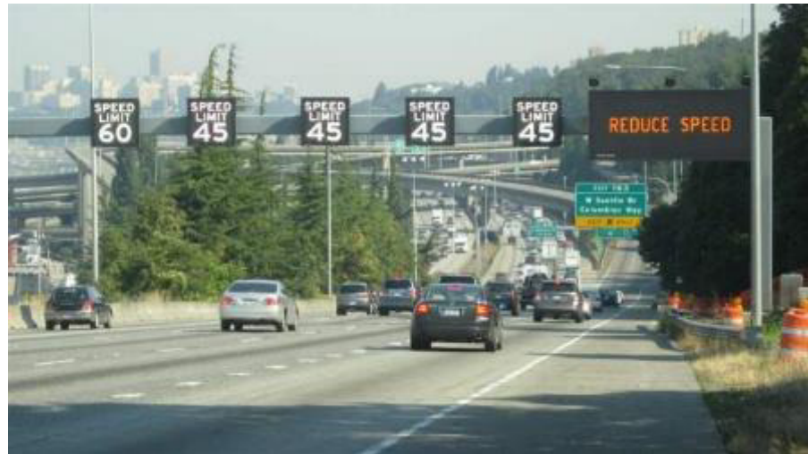
Figure 3.26. Variable speed limits on I-5 approaching Seattle in Washington.
