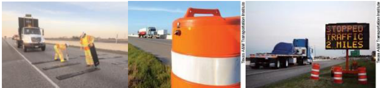
Figure 3.14. Texas Department of Transportation end-of-queue warning system consisting of (from left to right) portable rumble strips, speed sensor, and portable changeable message sign.
