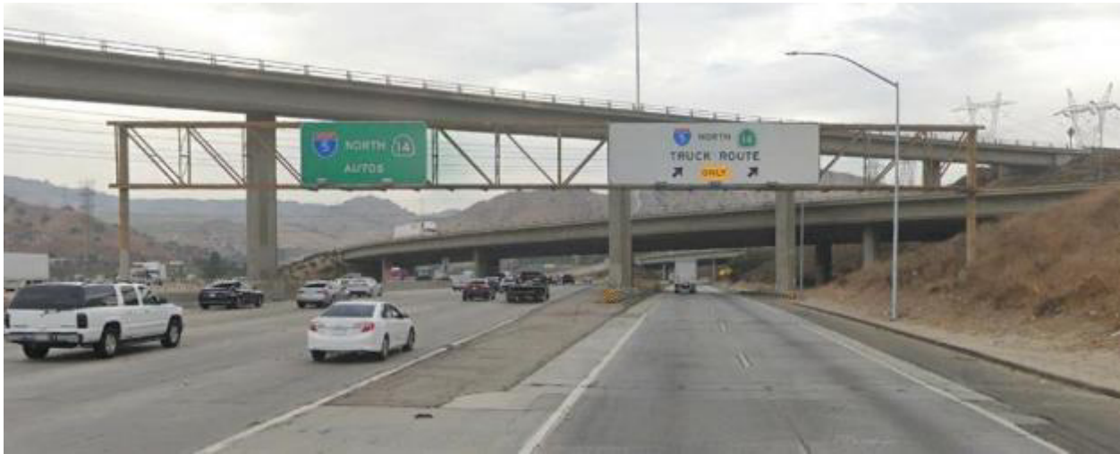
Figure 3.34. Truck-only lanes on I-5 in Los Angeles, CA.
