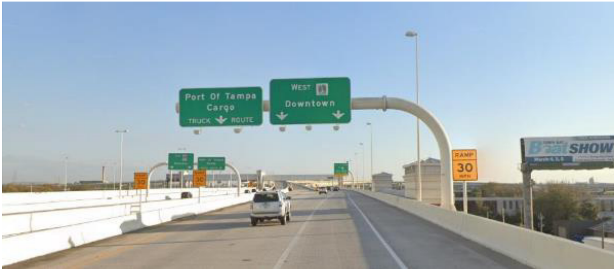
Figure 3.35. Port of Tampa truck access road.
