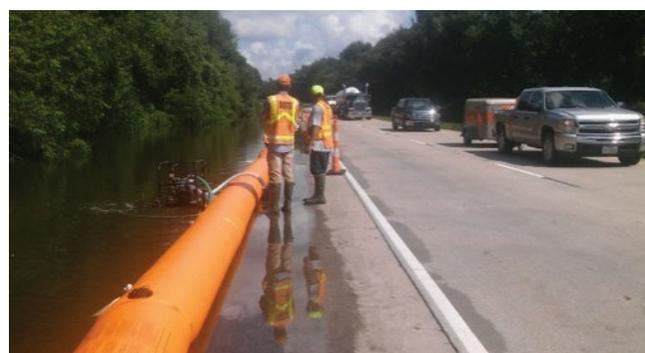
**Figure 1b.** The Louisiana Department of Transportation and Development (DOTD) checking water-filled barriers next to an evacuation route during March and August of 2019 flooding events. (Source: Louisiana DOTD)
