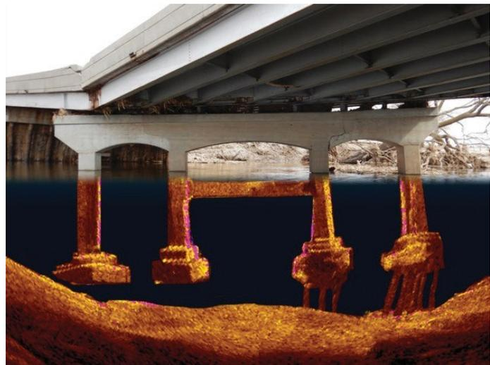
**Figure 4.** Underwater inspection of a Nebraska Route 13 bridge near Hadar included acoustic imaging that showed timber piles under the upstream footings were crushed or washed away. (Source: Nebraska Department of Transportation)
