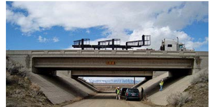
Photo Courtesy of FHWA
