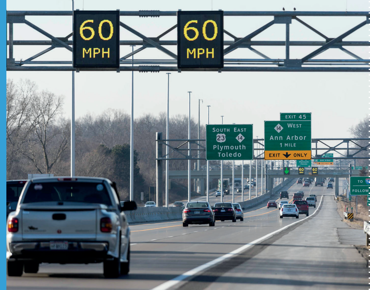
Michigan’s US-23 Flex Route, opened in 2017 north of Ann Arbor, utilizes active traffic management to address traffic, incident management, and motorist safety. Photo courtesy Michigan DOT
