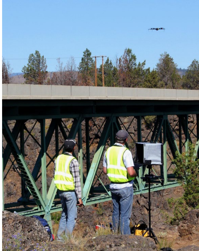
Figure 14. Photo. Unmanned aerial systems for construction inspection.
