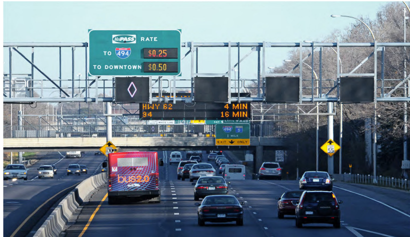
Figure 15. Photo. Signs for HOV lanes and general-use lanes side by side. (36) (Source: Minnesota Department of Transportation).
