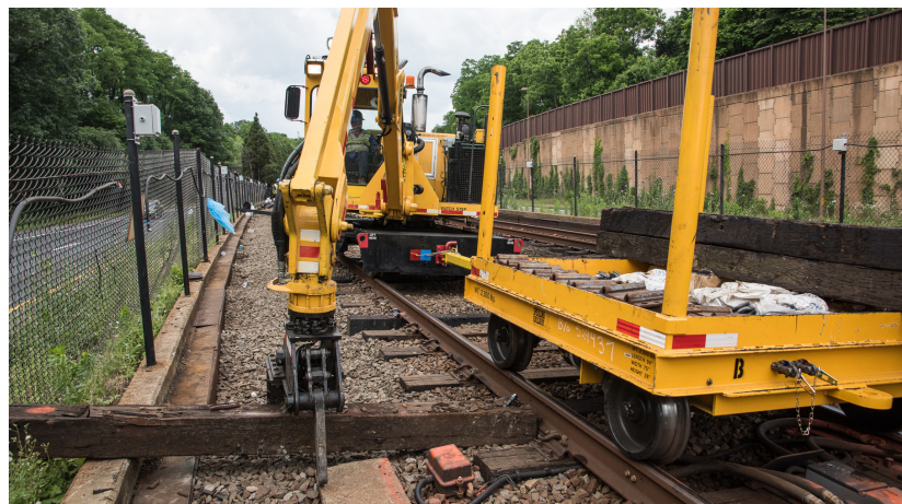
Figure 8. Photo. WMATA tie replacement during SafeTrack maintenance. (12) (Source: WMATA).
