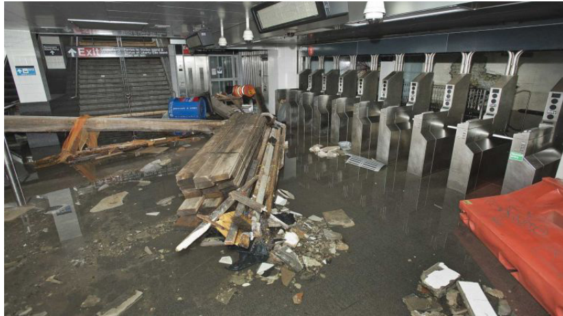
Figure 4. Photo. A subway station flooded by seawater during Hurricane Sandy (October 30, 2012). (3) (Source: Newsday/Metropolitan Transportation Authority/ Patrick Cashin).
