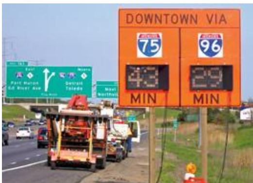
Comparative travel time displays in a Michigan work zone.
