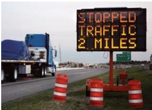
Portable queue detection and warning system upstream of a work zone in Texas.
