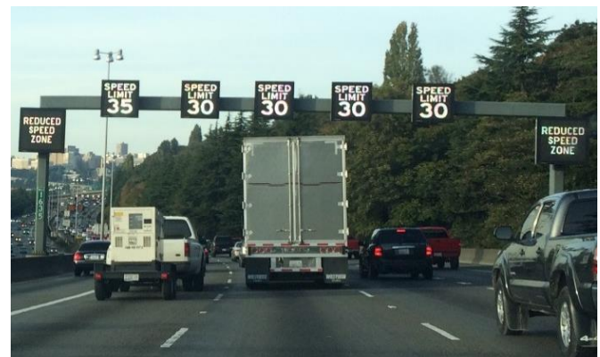
Lane control signs with variable speed limits were deployed near Seattle as a construction mitigation strategy.
