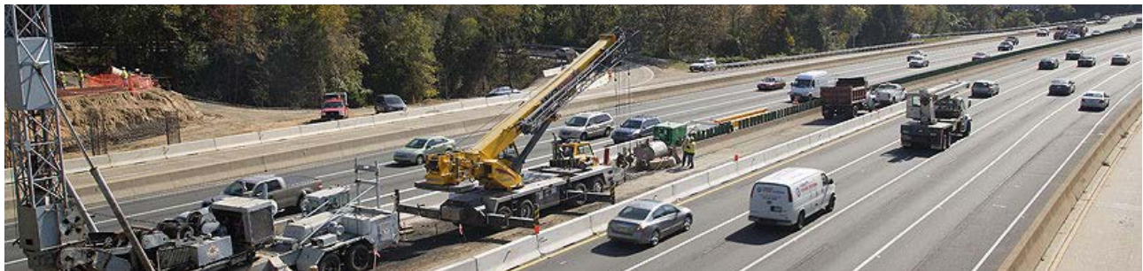
Figure 5. Photo. Construction of the I-495 Express Lanes in Northern Virginia.
