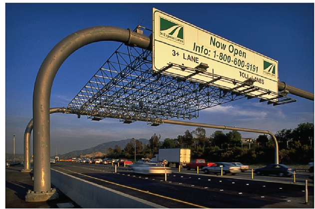
Transponders are read by overhead antennas, allowing tolls to be paid without stopping
