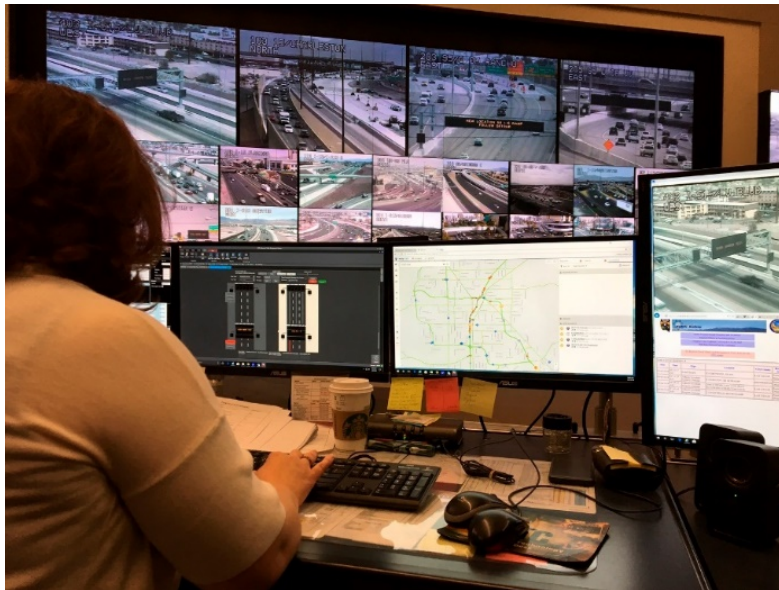
Figure 3. Photo. Traffic management center workstation at the Freeway and Arterial System of Transportation traffic management center, Nevada.
