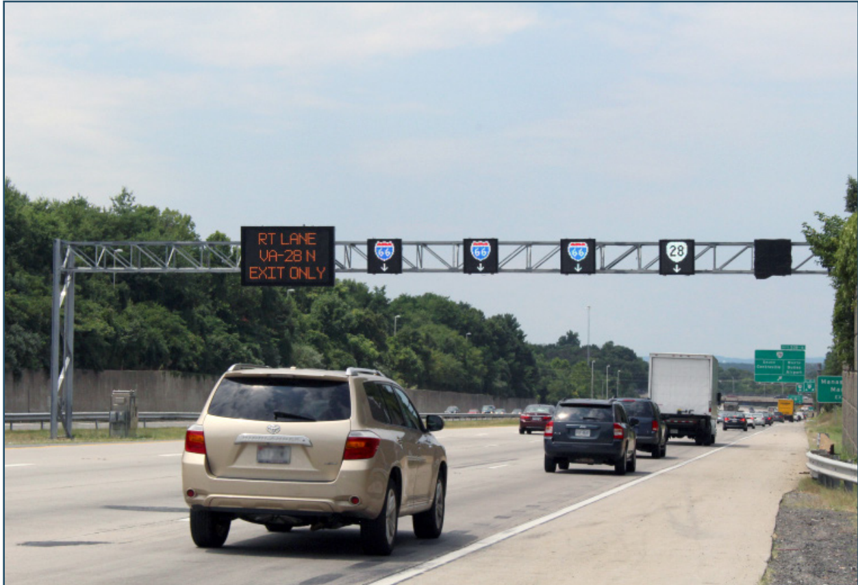
Figure 2. Photograph. Interstate-66 advanced traffic management including dynamic shoulder use.
