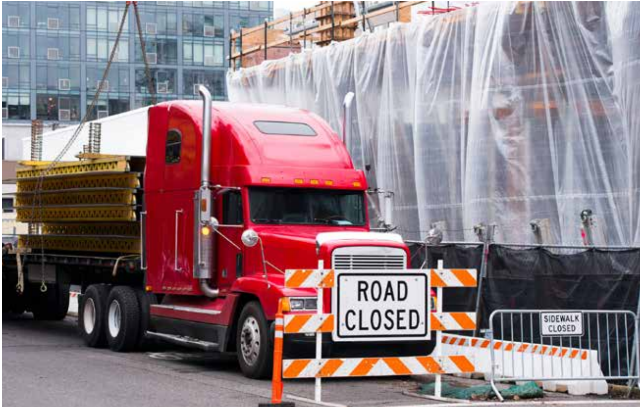
A truck being unloaded at an urban construction site. Source: 123rf.com.
