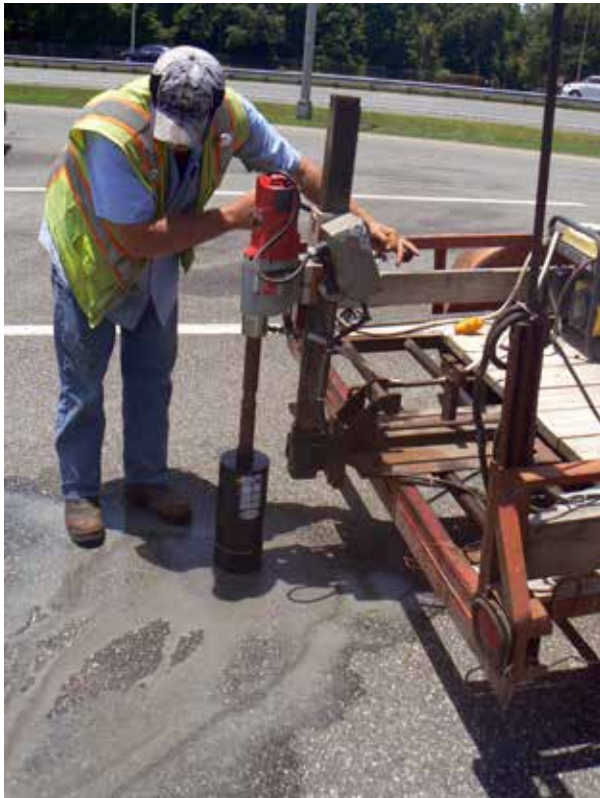
Installation of TPAS technology. Source: FDOT.
