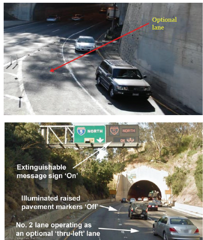
Figure 12. Photo. Ramp Configuration and Mainline Signage for Junction Control in Los Angeles, California.
