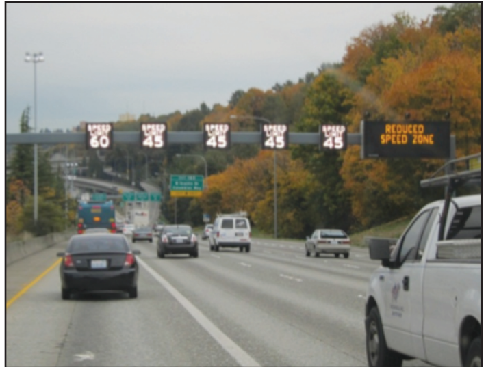
Figure 5. Seattle I-5 Northbound Active Traffic Management (termed Smarter Highways by WSDOT) – Source: Texas A&M Transportation Institute.
