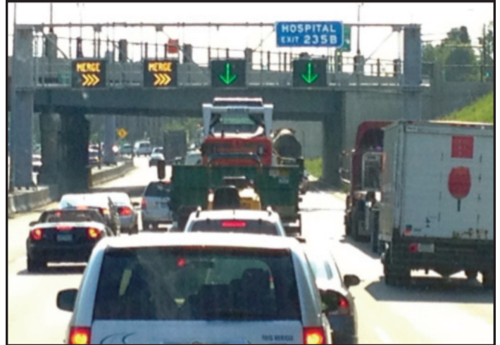
Figure 1. Minneapolis I-94 Westbound Active Traffic Management – Source: Texas A&M Transportation Institute.
