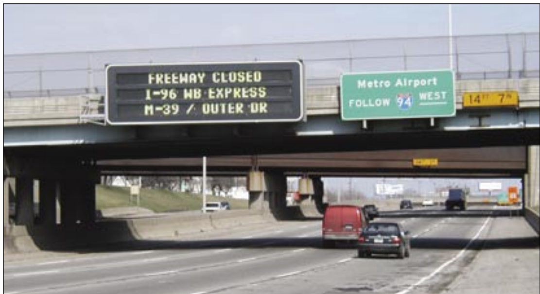
Figure 6-3. CMS informing drivers of a freeway closure
