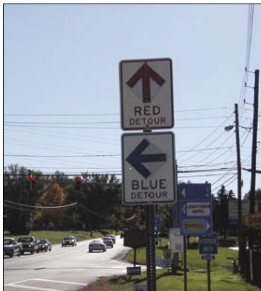
Figure 6-8. Color-coded alternate route trailblazer signs.
