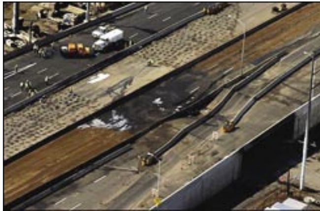
Figure 2-2. Buckling of I-95 due to tanker fire. (Source: Hartford Courant 11 )
