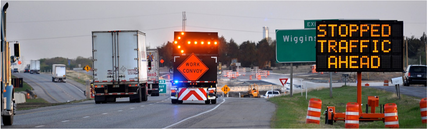
Figure 2. Safety contingency funds have been used for many countermeasures, such as for work zone intelligent transportation systems.
