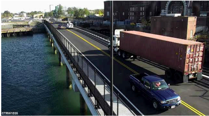
The dedicated freight corridor connecting the Port of Boston to I-93 opened in 2017. Source: Massachusetts Port Authority.
