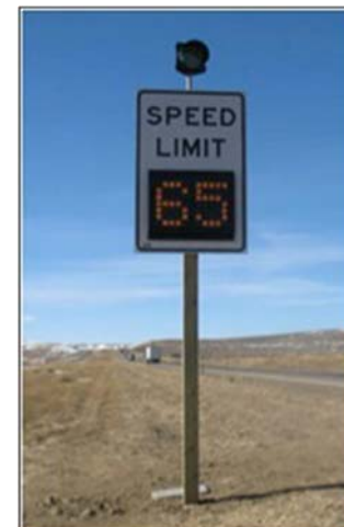
VSL on I-80, WY (Source: WYDOT).
