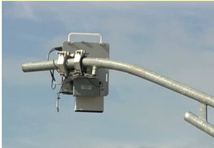
Figure 3. Photograph showing overhead antenna used in the SENTRI program (4).
